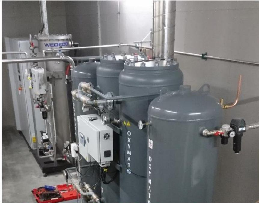
Figure 2.5 Full-scale installation of the ozonation system.
